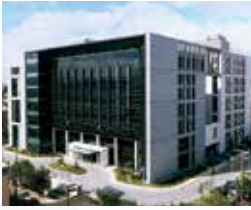
Taoyuan Technology Center (Green Building)
